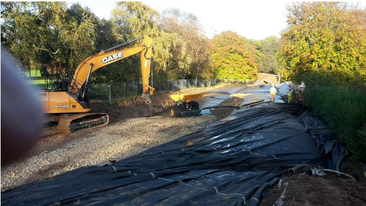
Geotubes full of silt
